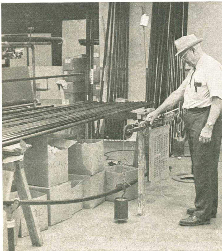
One of the many steps in the manufacture of fiberglass vaulting poles is determining the "flex" of the pole. A 52-lb. weight is hung on the pole half-way between two supports and the amount of deflection of the pole measured in inches. The further the deflection, the higher the number and the softer the pole. (Photo by George Moore)
